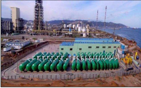
Figure 4: Station de dessalement Cap Djinet
